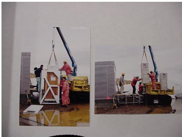
Carrying-in work of the hydrogen maser frequency standards in Summer Operation.
