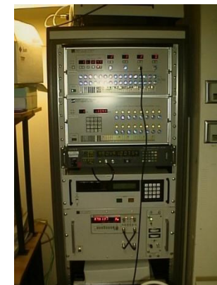
K4 back-end system installed in Syowa Station.
